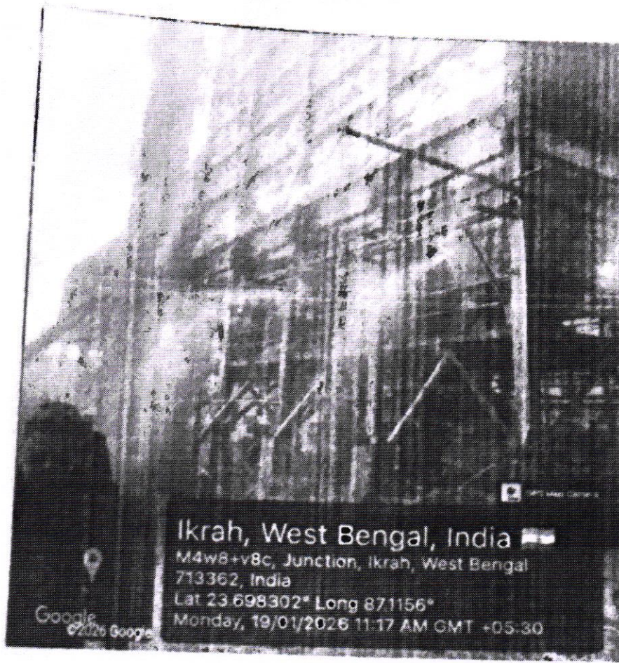
Only 04 nos of Fixed Type Sprinkler in operation at ESP of 1x350 TPD (Pic 3)
