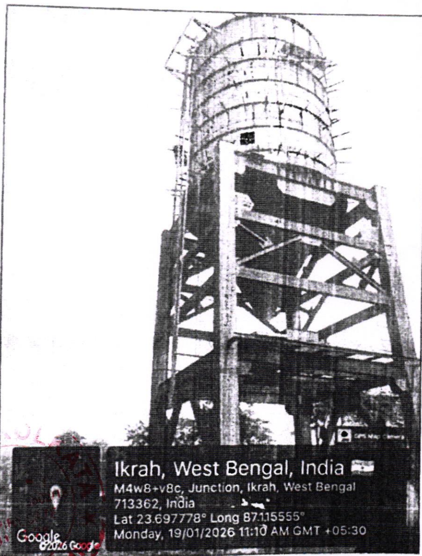
Ash silo not yet completed (Pic 2)
